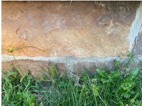
Stone foundation wall
