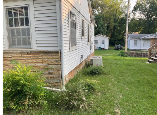
Right Side Grading
