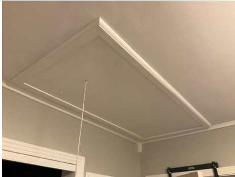
Attic Access Closed
