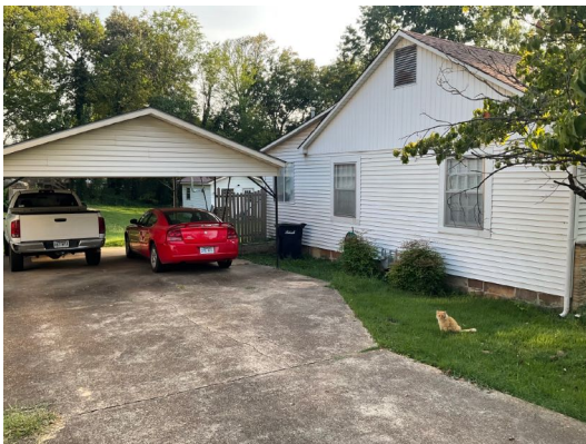
Left Side Grading
